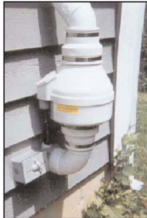
Example of a Depressurization System
