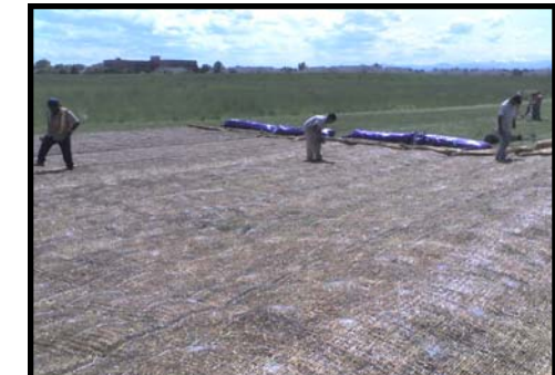
Repair to landfill drainage swale erosion mat
